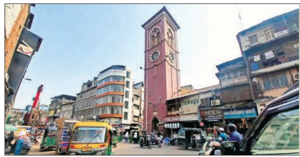
Provision made in municipal budget for repair, restoration of Clock Tower in Zampa Bazaar. HANIF MALEK
